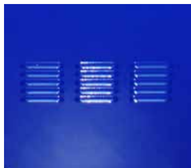
Louvers for Ventilation - Reduces Heat and Moisture
